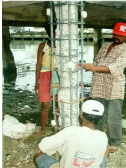
Fig. 7 Closer view of anodes installed
