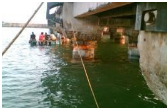
Fig. 4 Typical view of corroded member - Case 1
