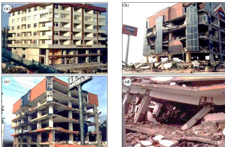
Fig. 1 Different levels of contribution of masonry infill walls to reinforced concrete frame responses: (a) limited masonry damage; (b) extensive damage to masonry, no apparent distress in frames; (c) total masonry damage with some distress in first-story columns; (d) total damage to masonry and structural collapse [1]
