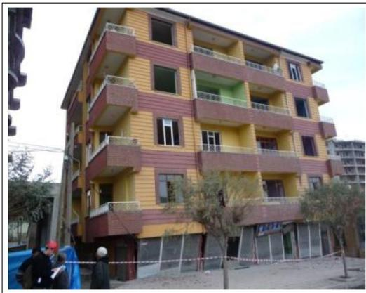
Fig. 2 A building after 2011 Van earthquake with heavy damage on first story walls [2]
