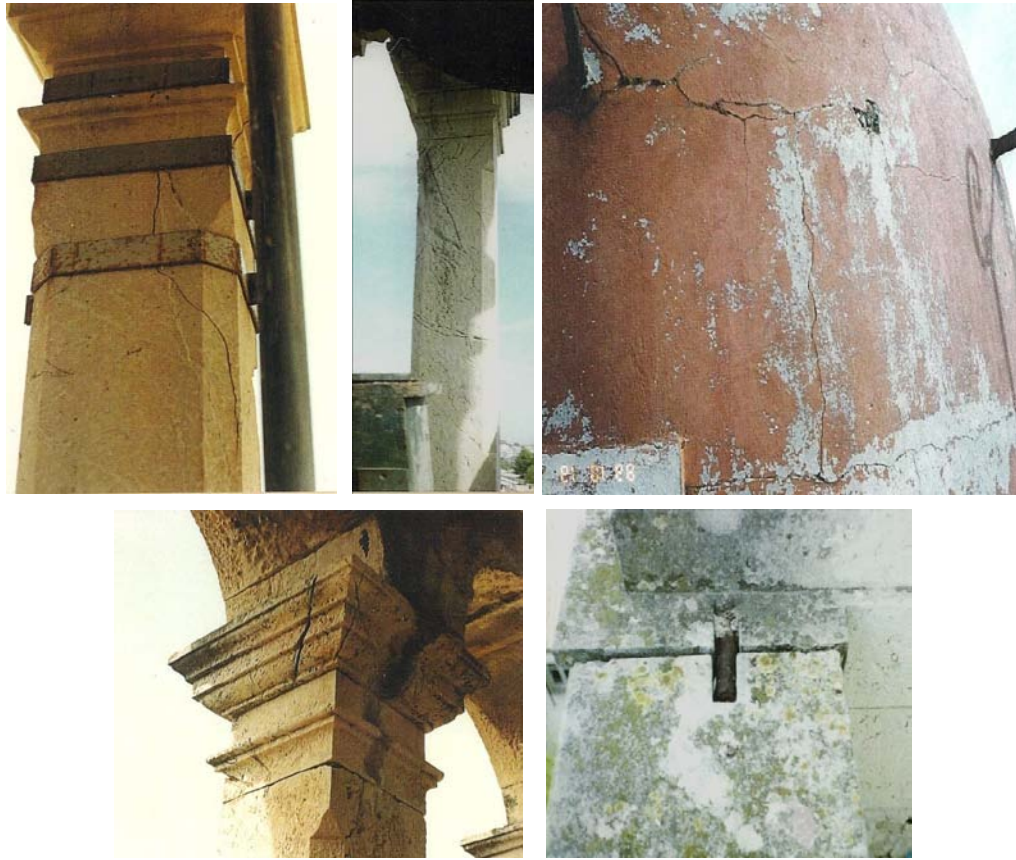
Fig. 2 Corfu bell-towers have suffered from damages and cracking from earthquakes
