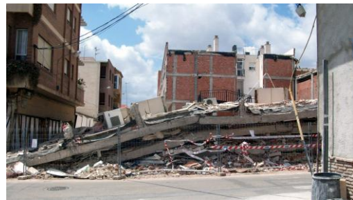
Fig.10 View from the main façade of the building that completely collapsed after the second event (Southern side)
