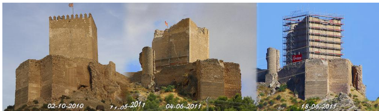
Fig. 2 Espolón Tower of the Castle ensemble, before and after the earthquake (left and centre), and under restoration (right). (Picture: Nandocd, www.flickr.com)
