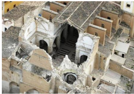
Fig.7 Church of Santiago in Lorca (Spain), after dome collapse and similar damage in the Duomo of San Massimo in L'Aquila (Italy) (Photographs: Atlas Agency, 201-05-13 and AP/Alesandra Tarantino, 2009-04-07)
