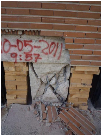
Fig. 16 Short column that did not collapse
