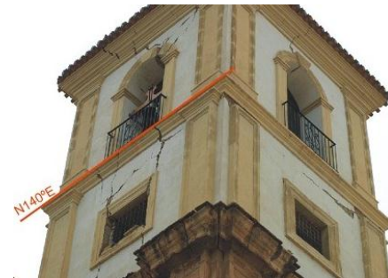
Fig.5 Damaged top of the tower, Church of Santiago (Scheme of the IGME Final Report)
