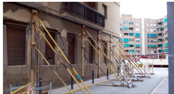
Fig. 18 Soft-story damage and scheme (P. Murphy) and induced short column by masonry walls (A. Aretxabala)
