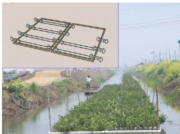
Fig. 6 Buoyant frame AFIs designed by Hubei University (Frame is of welded high-density polyethylene (HDPE) pipes filled with polyfoams)
