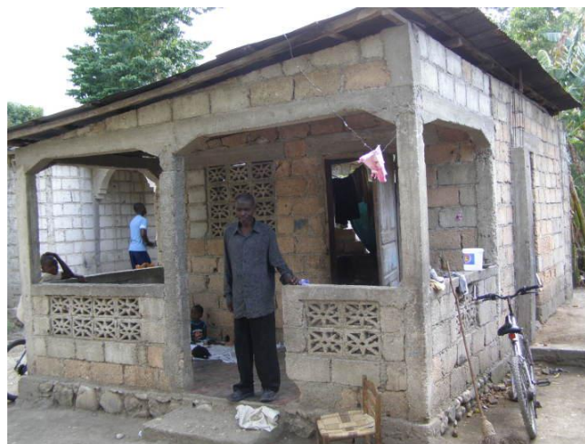
Fig. 22 Haitian example of CMU/captive masonry construction
