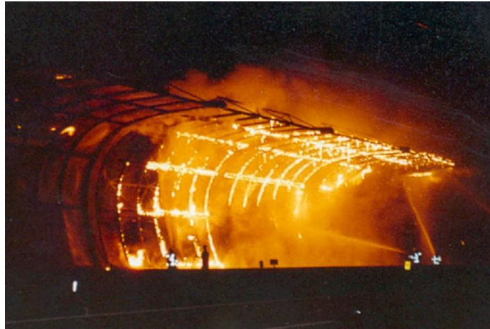
Fig. 11 “Incombustible” acoustic screen along the A16 highway near Dordrecht on fire (May 08, 2001)
