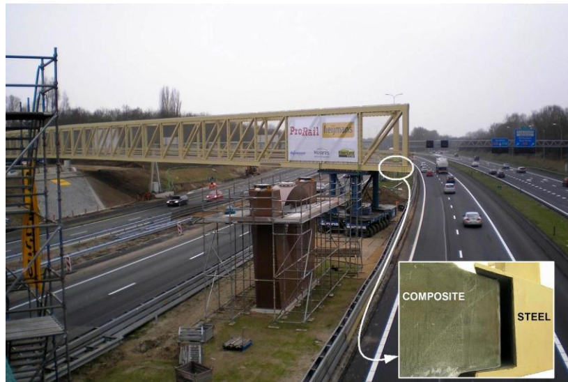
Fig. 6 Launching of a viaduct with composite deck (supplied by FiberCore Europe) over the A27 highway nearby Utrecht, the Netherlands [11]
