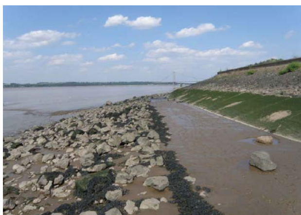
Photograph 2 Foreshore at Barton on Humber in which the toe of the sea wall has been extended in response to foreshore lowering. Debris from previous rock armour lies on the upper foreshore
