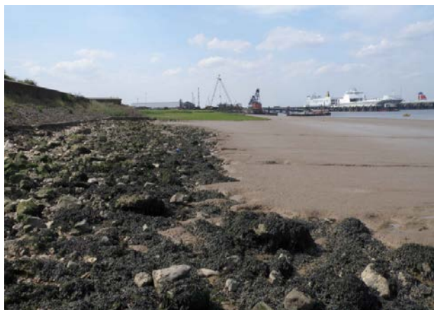
Photograph 1 Foreshore at North Killingholme depicting lowered mudflats in front of the sea wall which is partially protected by debris from previous rock armour
