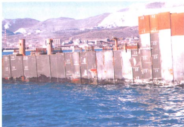
Figure 2. incline of the segment of the sheet-pile after storm
